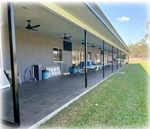
2021 – new tiles have been laid on front veranda
